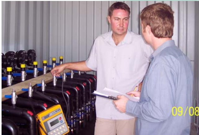
Gas manifold station / gas well on site
