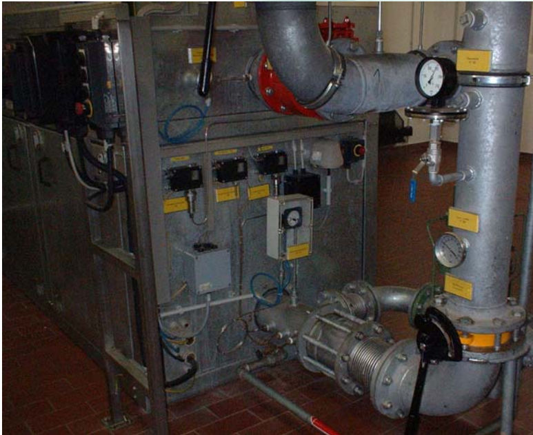
Booster station: „EX“ and „Normal“ but gas tight
